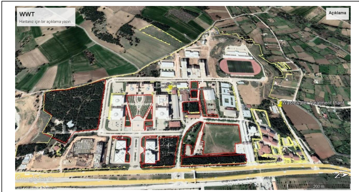
Wastewater treatment plant location
